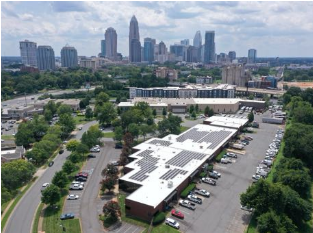
Pictured: City of Charlotte Spratt Street Facility, Charlotte, North Carolina; 243 kWdc
