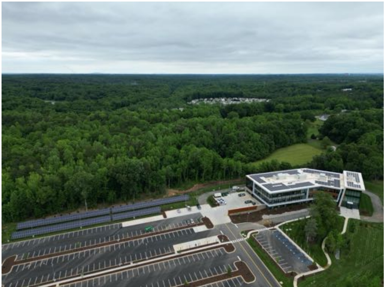
Pictured: Continental Tire Headquarters in Fort Mill, South Carolina; 357 kWdc
