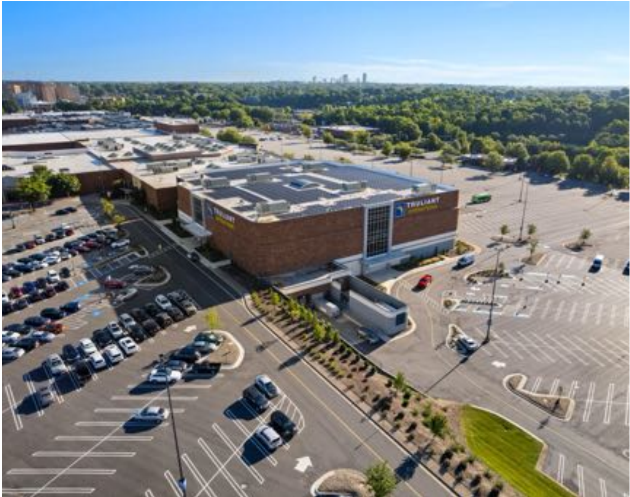
Pictured: Truliant Operations Center in Winston-Salem, North Carolina; 352 kWdc
