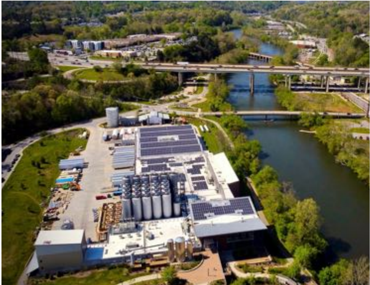
Pictured: New Belgium Brewing in Asheville, North Carolina; 446 kWdc
