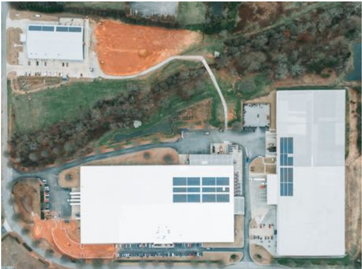
Pictured: Takeuchi Headquarters in Pendergrass, Georgia; 810 kWdc
