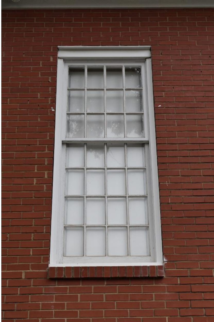
Typical twelve-over-sixteen wood sash window
