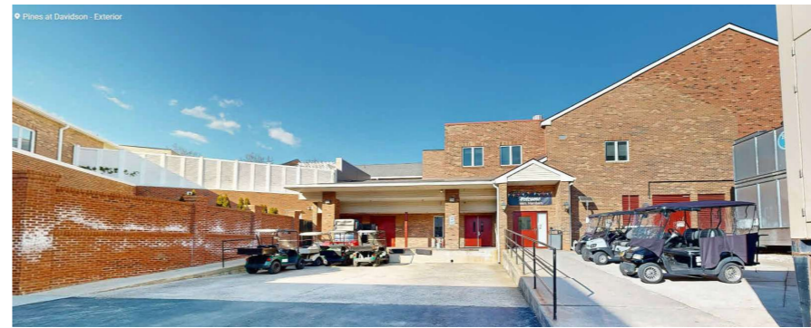
C. COMMONS BUILDING LOADING DOCK
