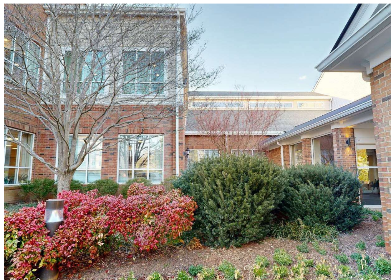
EXISTING CONDITIONS (PHOTO)
