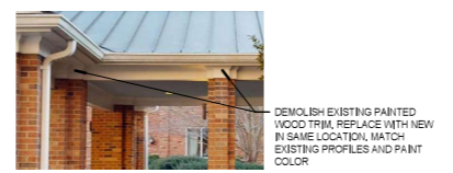
EXISTING CONDITIONS EXISTING VESTIBULE EXTERIOR
