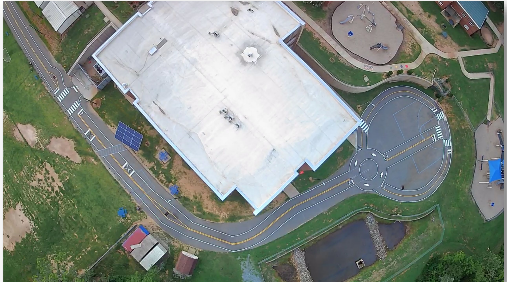
Drone image from RAM Pavement
