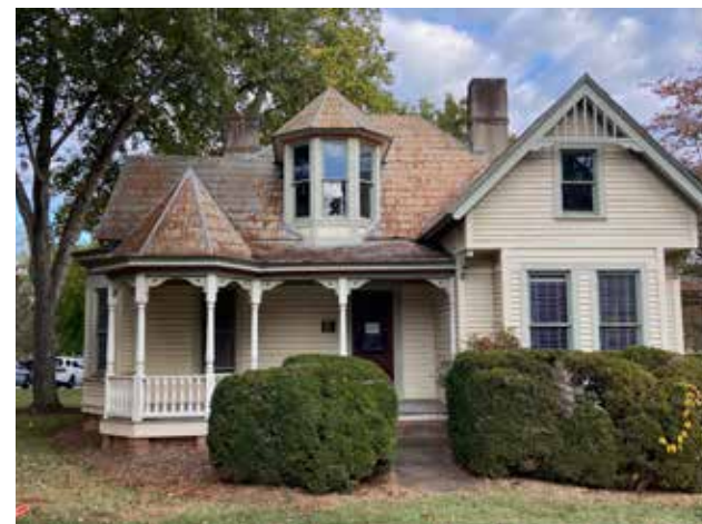
This Queen Anne example has a wide variety of wood details in the gable end and on the porch.
