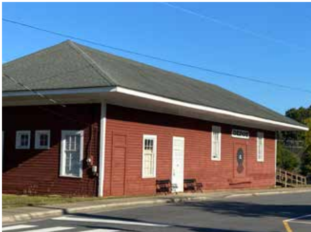
The historic depot building is wood frame with wood siding, trim, windows and doors.
