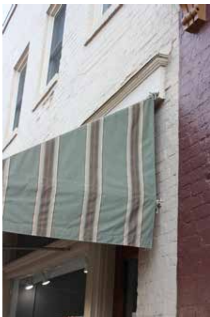
A simple metal frame with hooks on the storefront support this non-operable awning. Any attachments to brick must be made in the mortar joint to avoid damage to the brick.
