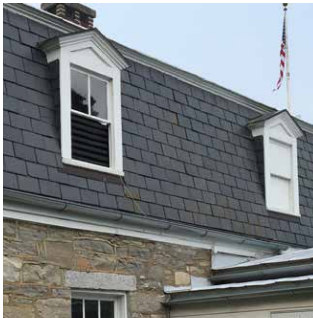
An example of a ventilated window on mothballed vacant historic building.
