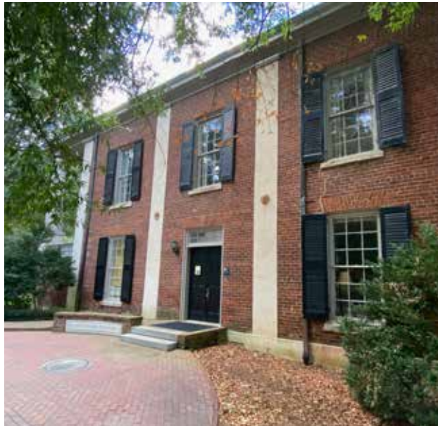
Stucco is used for details, such as pilasters, columns, and gables on these Davidson College buildings.
