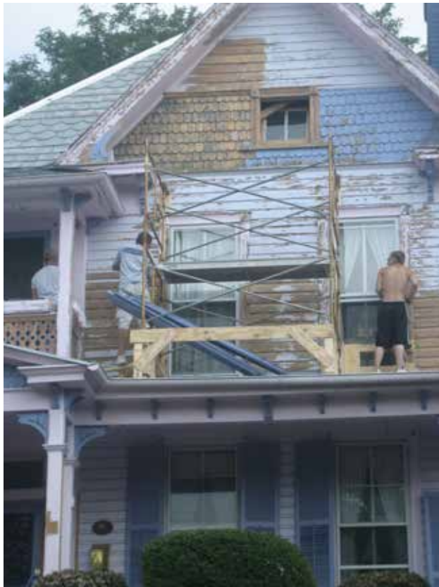
This photo shows the comprehensive preparation needed when the existing paint has failed and is peeling. In those cases, the original paint should be carefully removed to the original wood before being repainted.
