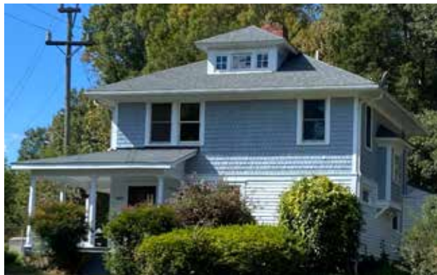
There is a wide variety of wood frame houses in the historic district with details ranging from simple lap siding to decorative shingles and trim.
