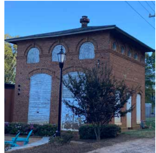
An example of a vacant building in the Davidson historic district that appears well secured.
