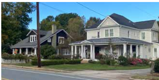
Roofs in the historic district range in character, shape, and original materials as seen in these two photos. Roof types may include gable, hipped, shed, along with variations and combinations of all of the above.
