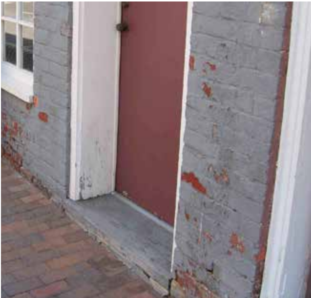
Rising damp from the ground below can saturate brick and cause paint and mortar failure.
