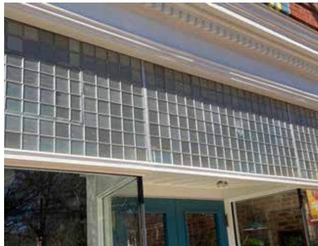
Prism glass was often used in transom windows on commercial buildings. The glass diffuses the light entering the interior space.
