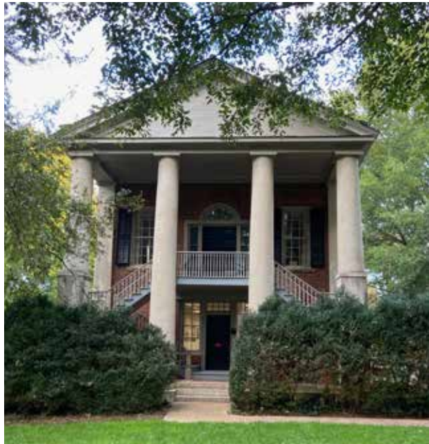
Stucco is used for details, such as pilasters, columns, and gables on these Davidson College buildings.
