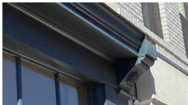
Metal cornices are very common on commercial historic buildings.
