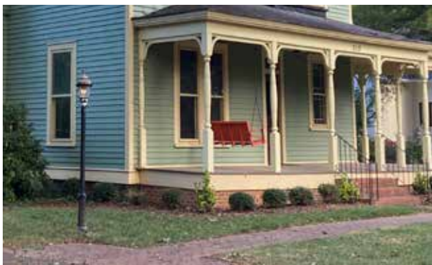
Brick foundations are typical on Davidson's historic frame residences as shown above and below.
