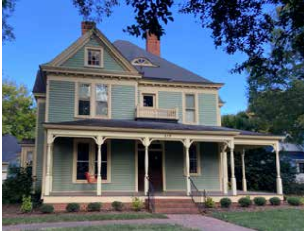
A Queen Anne house with a decorative wrap-around porch.
