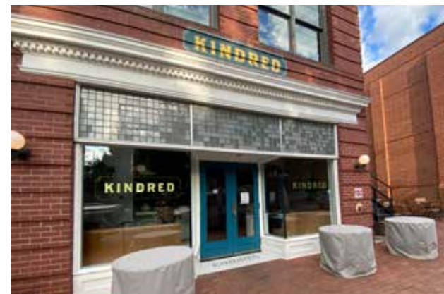
The original prism glass transom is a rare survivor of this original storefront and adds historic character to the building's facade.
