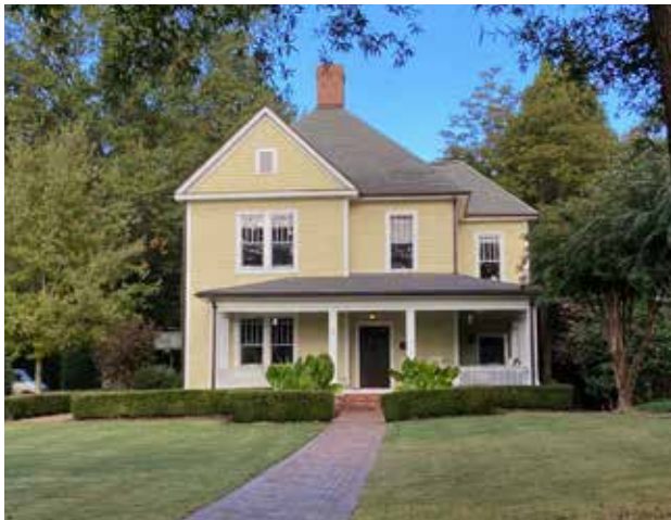
559 N. Main Street is a two-story Queen Anne dwelling with its asymmetrical facade, complex roof with gable and hipped forms, paired windows, and full-width front porch.
