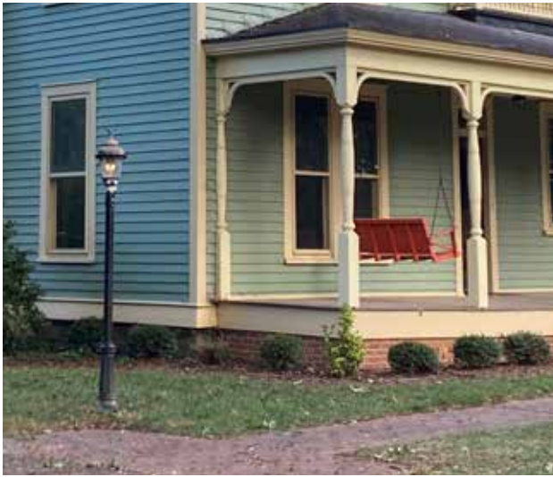
Many residential buildings have pole lights to illuminate the sidewalk to the front entrance.
