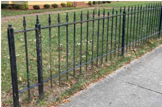
Metal picket fences are located on some historic residential sites.
