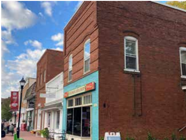
The majority of downtown commercial buildings are brick masonry construction.
