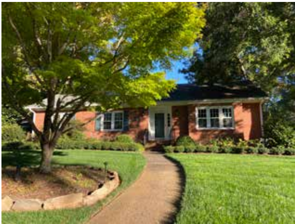
139 Woodland Street is a Ranch house example with its simple one-story design executed in brick veneer, with multiple windows
