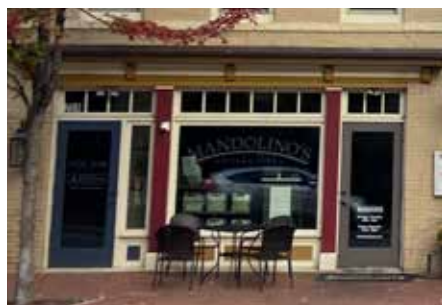
This well designed storefront retains its upper story entry, its transom and its paneled bulkheads.
