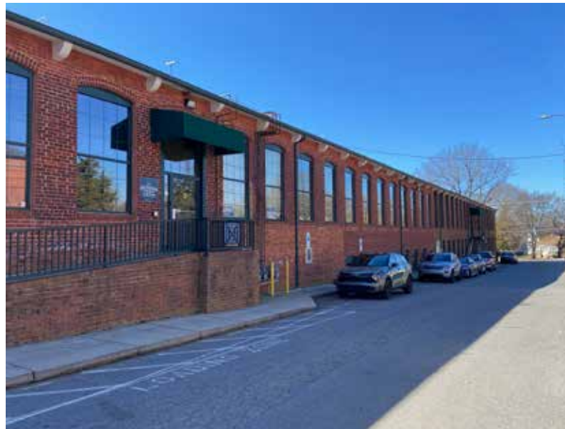
This brick industrial building on Delburg Street, formerly the Delburg Cotton Mills, has been adapted to new uses. Its large scale, single story, and rows of large double-hung windows reflect its original design that related to its original function as a mill.
