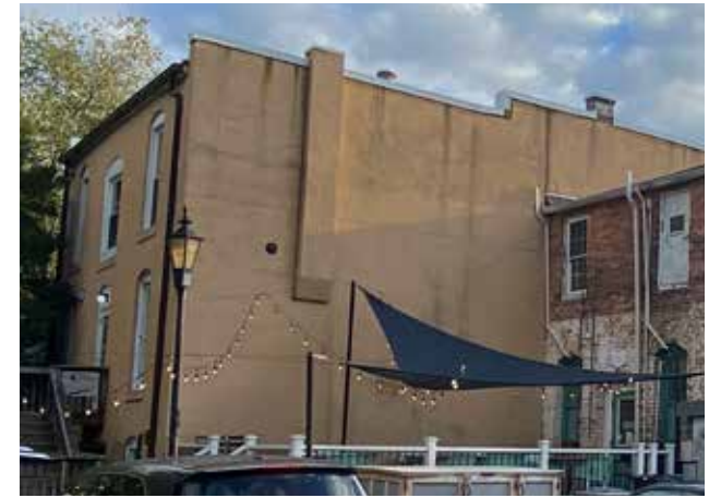
Stucco is also found on side elevations of historic downtown buildings in Davidson.
