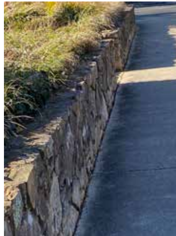
Stone retaining walls are also a feature found throughout the district.
