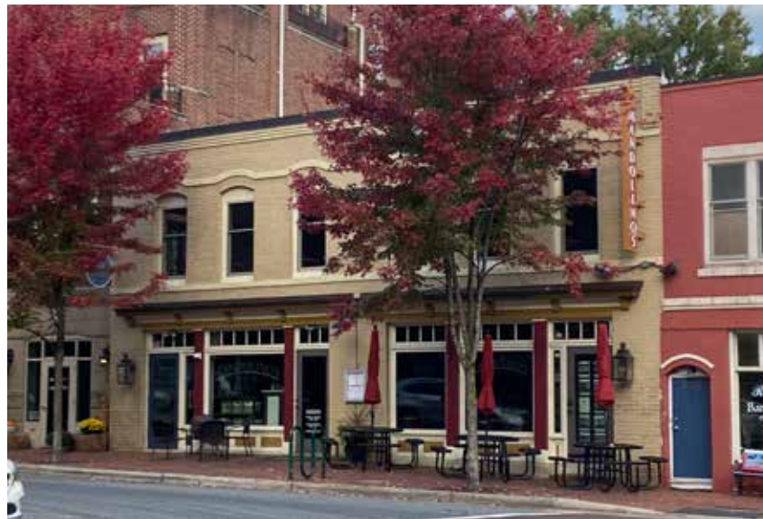
Two-story commercial buildings may have decorative cornices at the roofline and at the storefront. They also may have surviving transoms above the display windows and a second entry door for access to upper floors.
