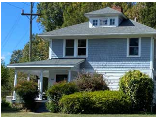
This foursquare house example has wood shingles and siding and simple wood trim.
