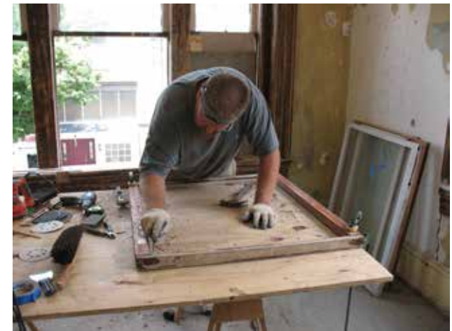
It is important that the selected contractor has specialized experience in working on historic buildings as in this photo of a historic window being repaired instead of being replaced.
