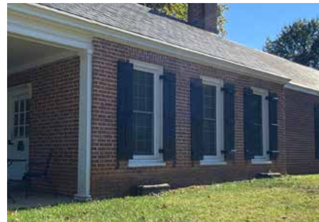
Brick buildings typically have brick continuing to the foundation and if it extends from the building's wall, it is known as a water table .
