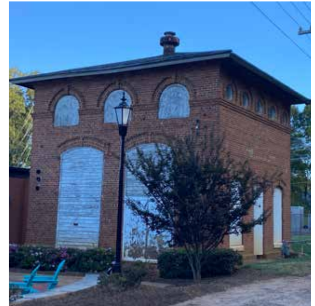
An example of a vacant building in the Davidson historic district that appears well secured.
