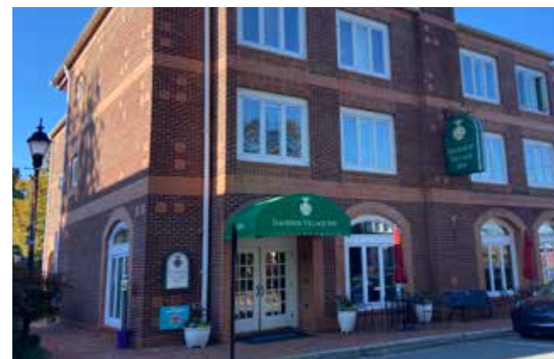
This curved awning is a good example of fitting the awning to the arched opening.
