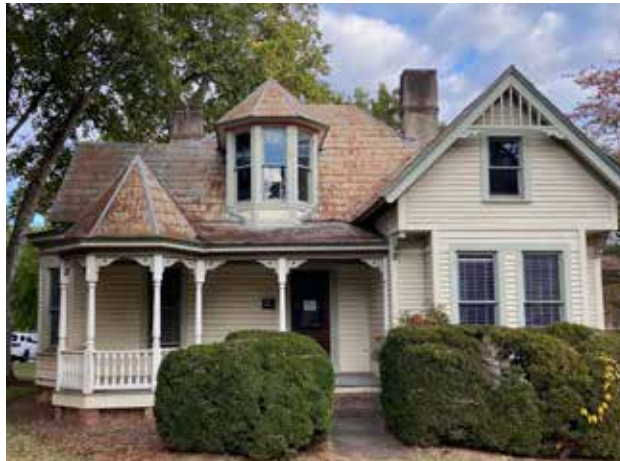
Metal shingle roofs are still intact on some historic houses in the district. This handsome example shows the need for maintenance and repainting.
