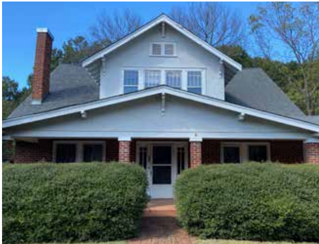
Stucco is used on many historic houses in the district such as this bungalow example.
