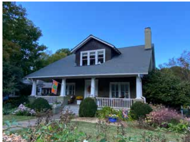
623 N. Main Street is a bungalow dwelling with its prominent gable roof containing a large three-windowed dormer and extending over the full width porch below.
