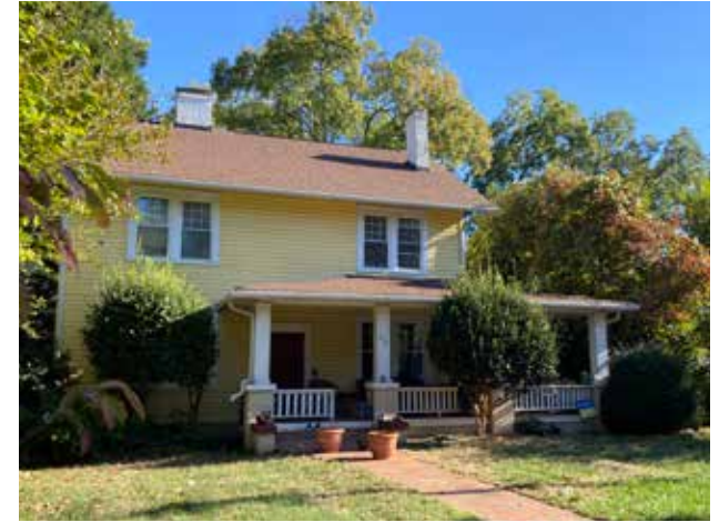
An example of a stretched Four Square style dwelling with an asymmetrically placed porch.
