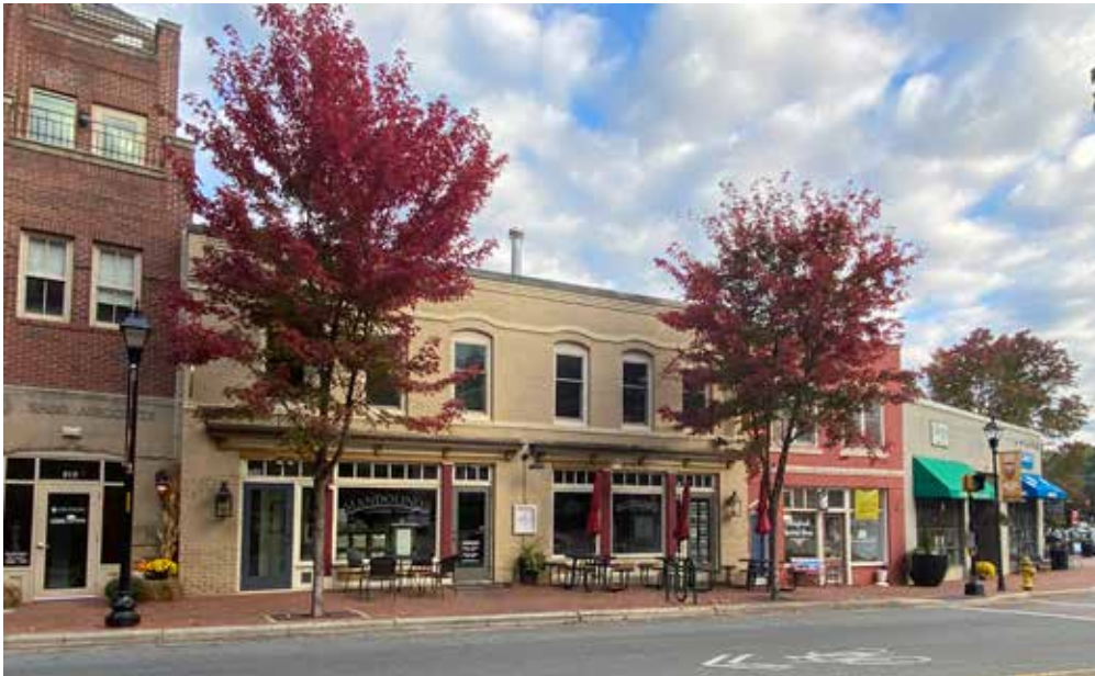
Davidson's Main Street is inviting and well maintained. Recently, existing buildings have been rehabilitated and new commercial buildings have been added that complement the historic district character.
