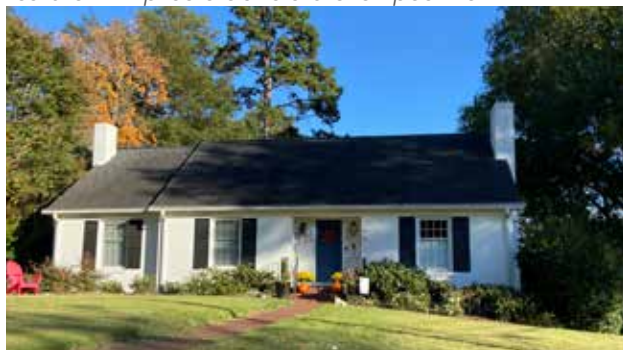
321 Woodland Street is a one-story brick Colonial Revival house with end chimneys and recessed entry.
