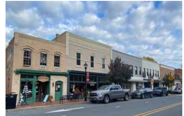
Commercial downtown buildings in the historic district typically have zero front setback and no site elements.
