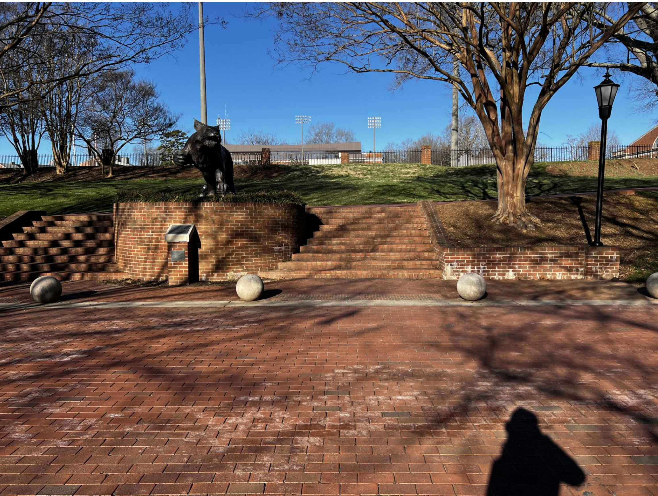
ADDITION VIEW FROM BAKER DRIVE
