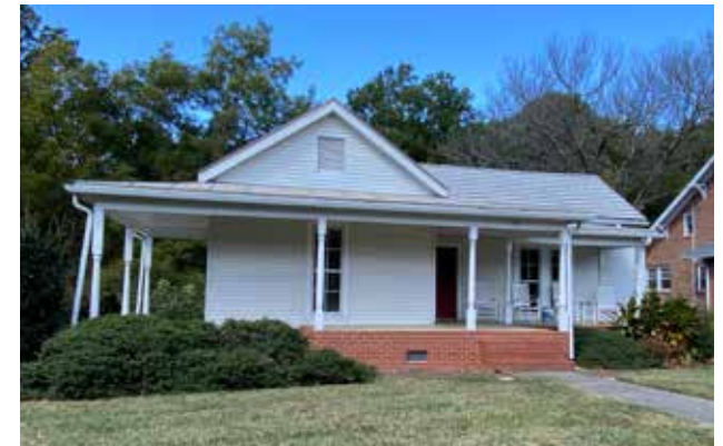
705 N. Main Street is a simple frame house in the local district that has an "L" shaped plan with intersecting gable roofs and a full-width wrap around porch supported by turned posts.
