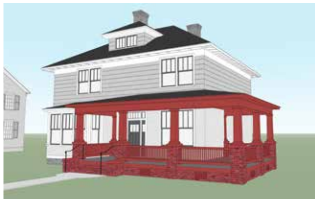
Foursquare houses in Davidson feature asymmetrical full porches.
