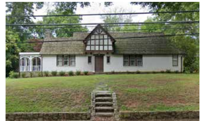
838 Concord Road has Tudor Revival details with its timber-framed entry gable flanked by small casement windows along with sets of triple windows.
