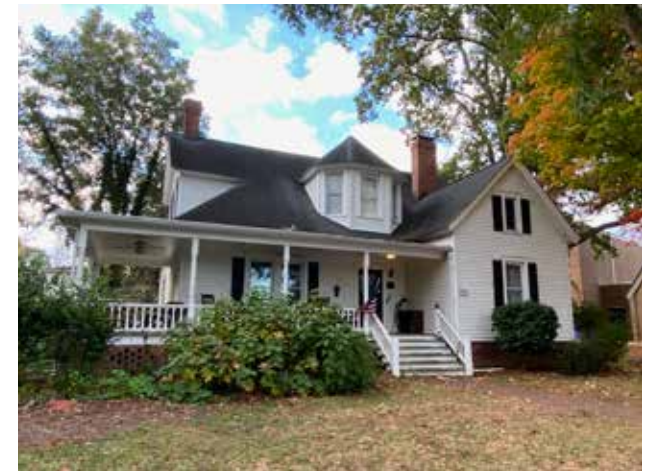
223 S. Main Street is a one and one-half story Queen Anne style house with its large bay window dormer, side and end gable roof forms, wraparound porch with turned columns and tall chimneys.
