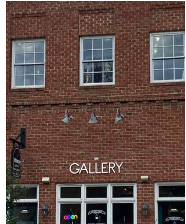
Besides public streetlights, some commercial buildings have shielded facade lights to light entrances.
