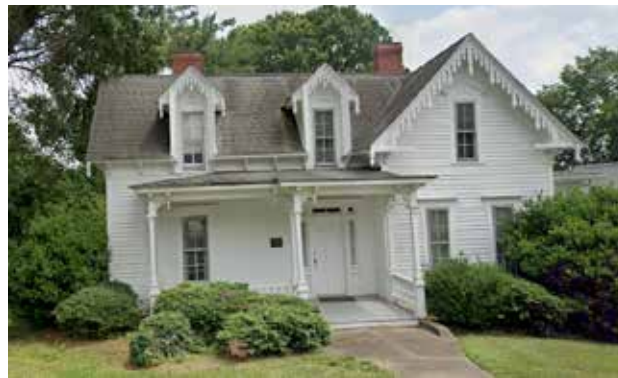
305 S. Main Street is a fine example of the Carpenter Gothic with its decorative wood details on the gable bay and the two gable dormers.
