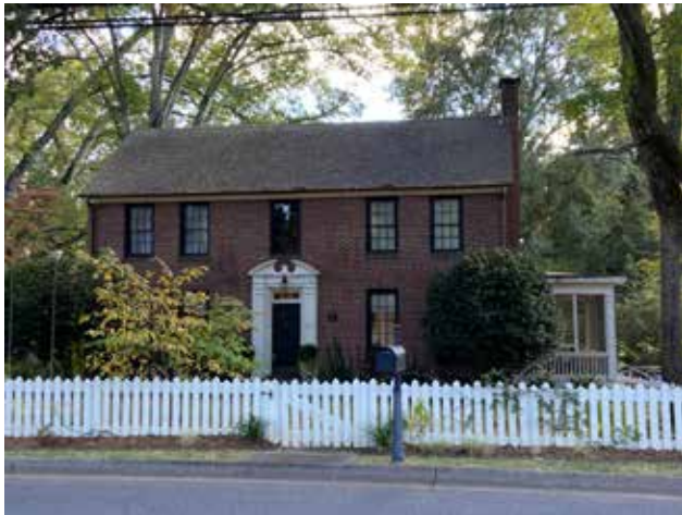
Wood picket and board fences are found throughout the district.
