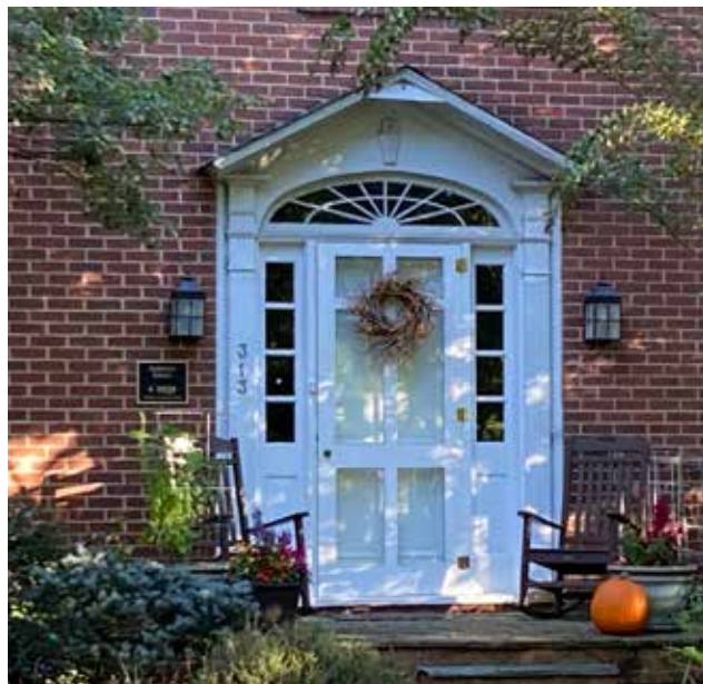
This six-paneled storm door was designed to match the divisions of the six-paneled door behind it.
