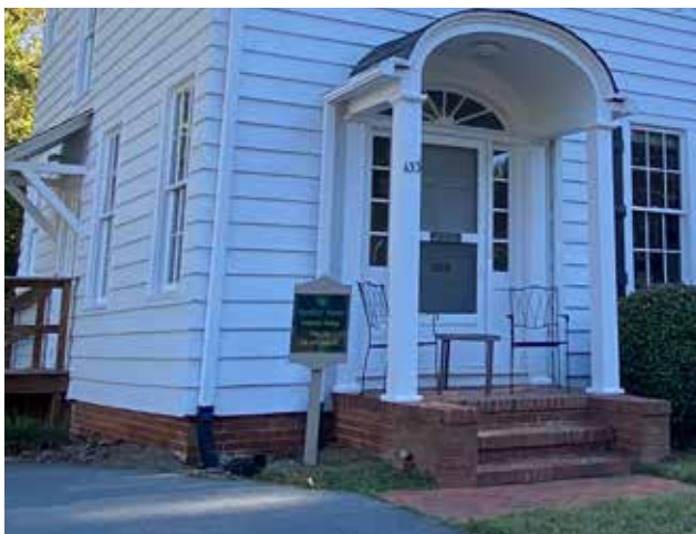
Brick foundations are typical on Davidson's historic frame residences as shown above and below.
