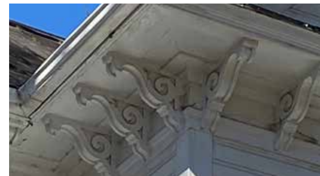
Queen Anne and Italianate buildings can have deep cornices with highly decorative carved brackets.
