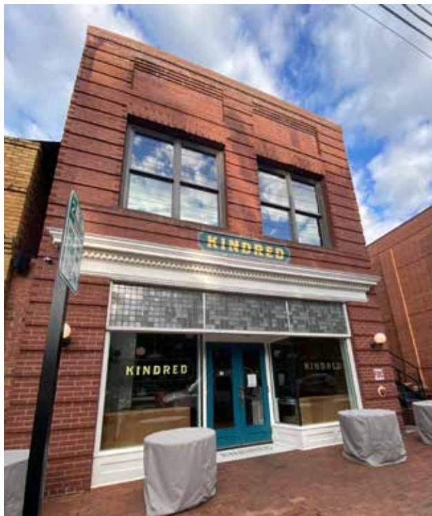
Brick buildings can have a variety of details such as recessed panels, a corbeled cornice and end quoins.
