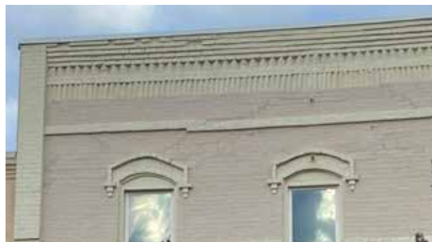
This brick cornice has a variety of brick configurations.
