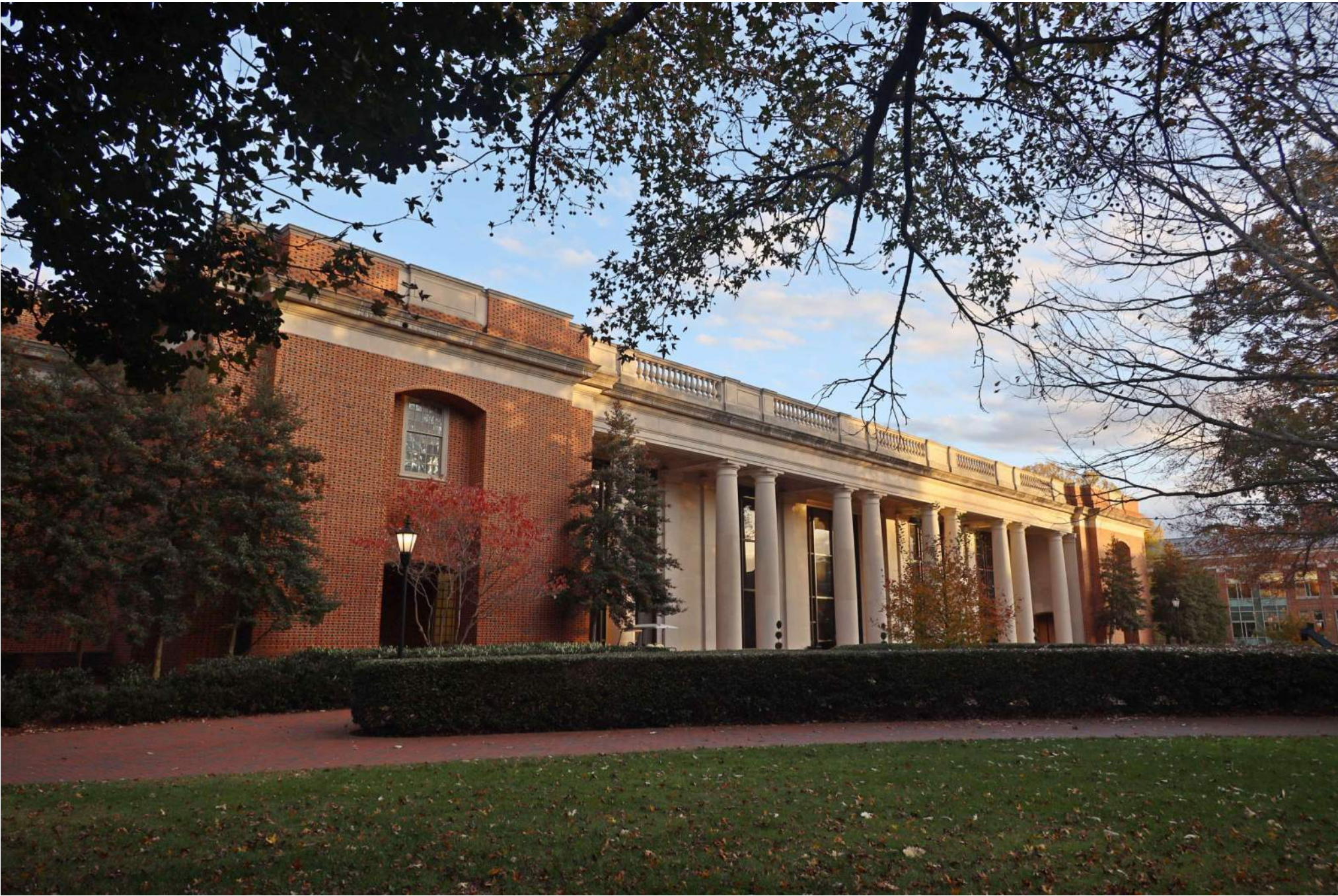
WEST APPROACH 1 - EXISTING
