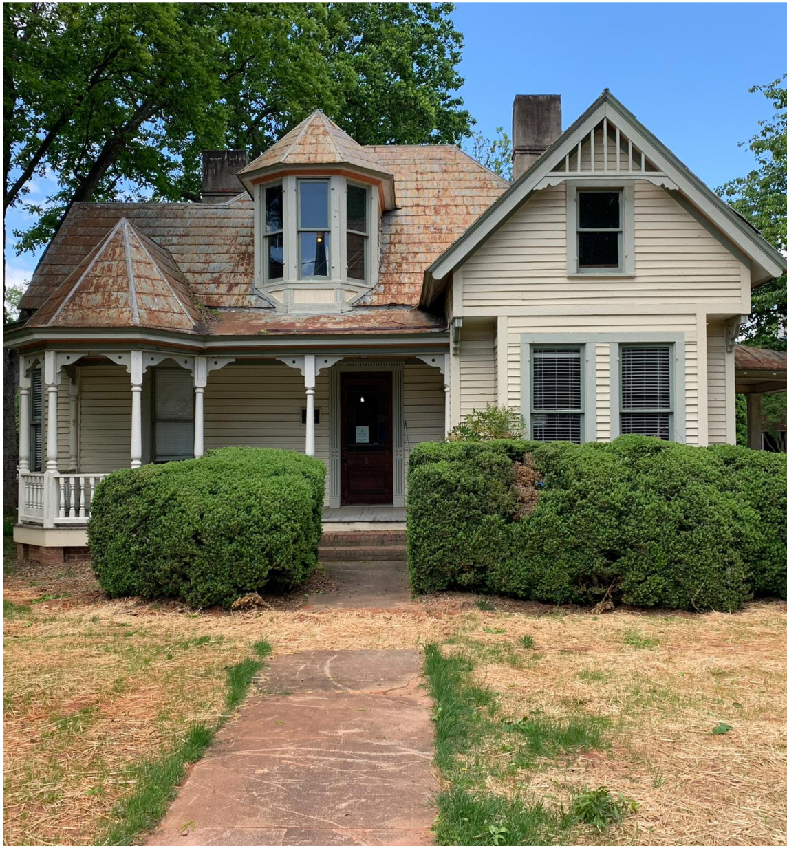
Figure 1. Sloan House Front Facade
