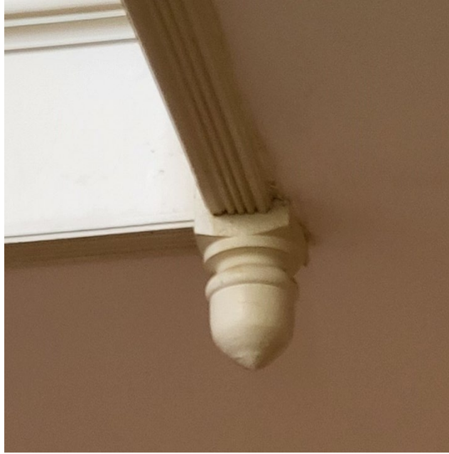
Detail of acorn-shaped pendill and molding in first floor stair hall (above) and detail of balustrade and newel (below). The glass paned door in the image below leads to the living room. The six panel wooden door in the background is the main entrance.
