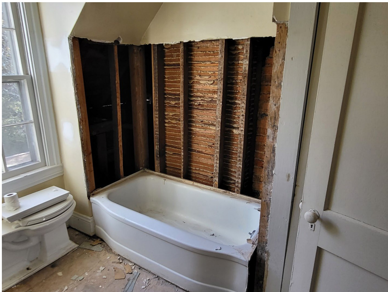
Second floor bathroom, wood lath and plaster wall system (above). Illustrative examples of door hardware typical throughout the house (below).
