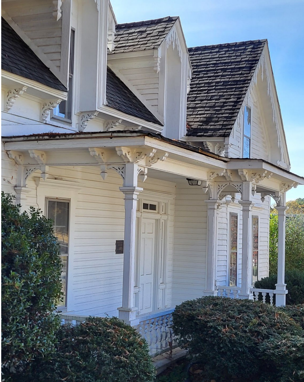
Front porch and main entrance.
