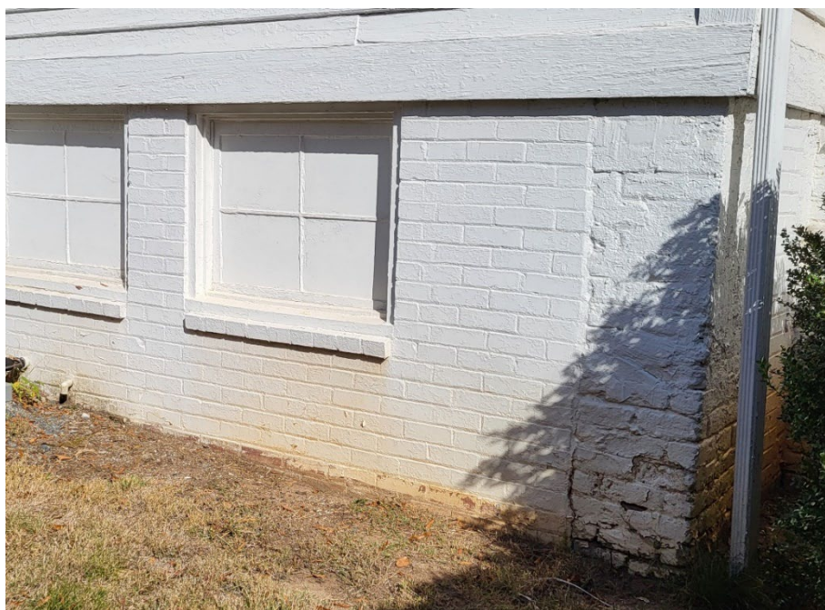
South elevation foundation.
