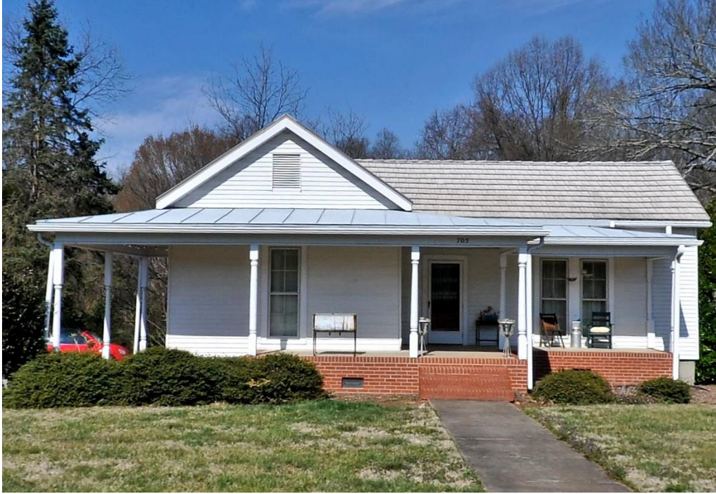
Figure 1. 705 N Main Street - Front Facade
