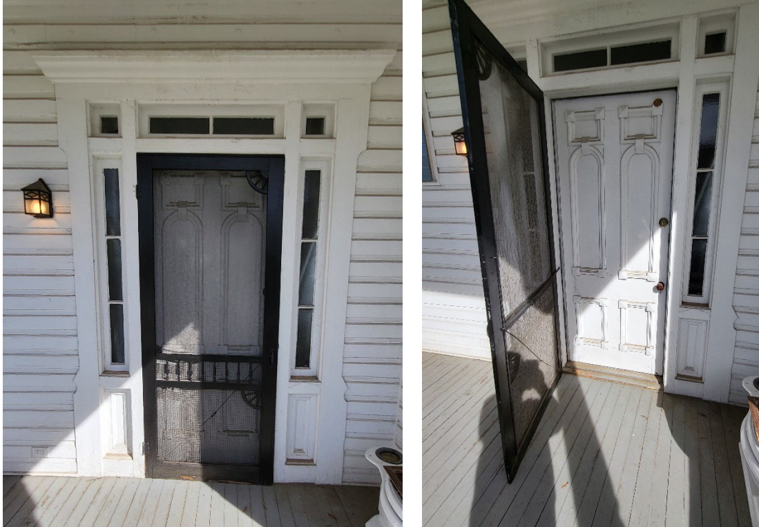
South elevation entrance.
