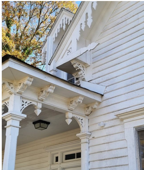
Detail of decorative sawnwork and pendills on front elevation of Brattain House.
