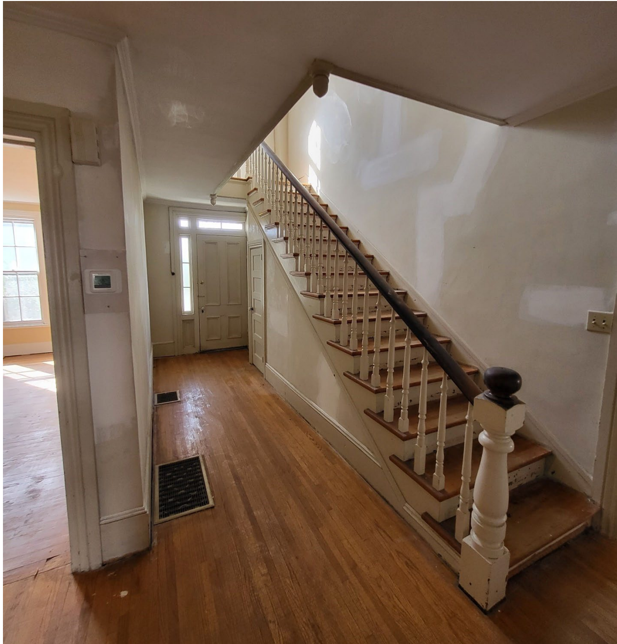
First floor stair hall and stairway. The doorway in the left foreground leads to the den. The door in the rear center is the south elevation entrance; to its right is the powder room door. Picture also shows illustrative original wood floors and crown and baseboard moldings typical throughout the house, as well as the acorn-shaped pendills.
