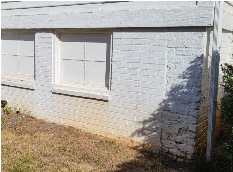
South elevation foundation.
