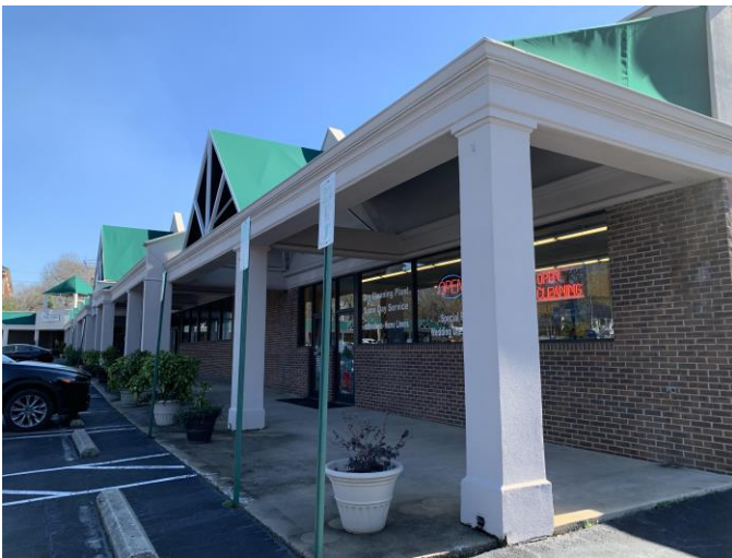
Figure 3. Existing Facade Details
