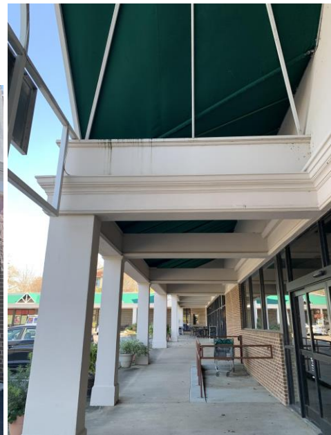
Figure 4. Existing Facade Details
